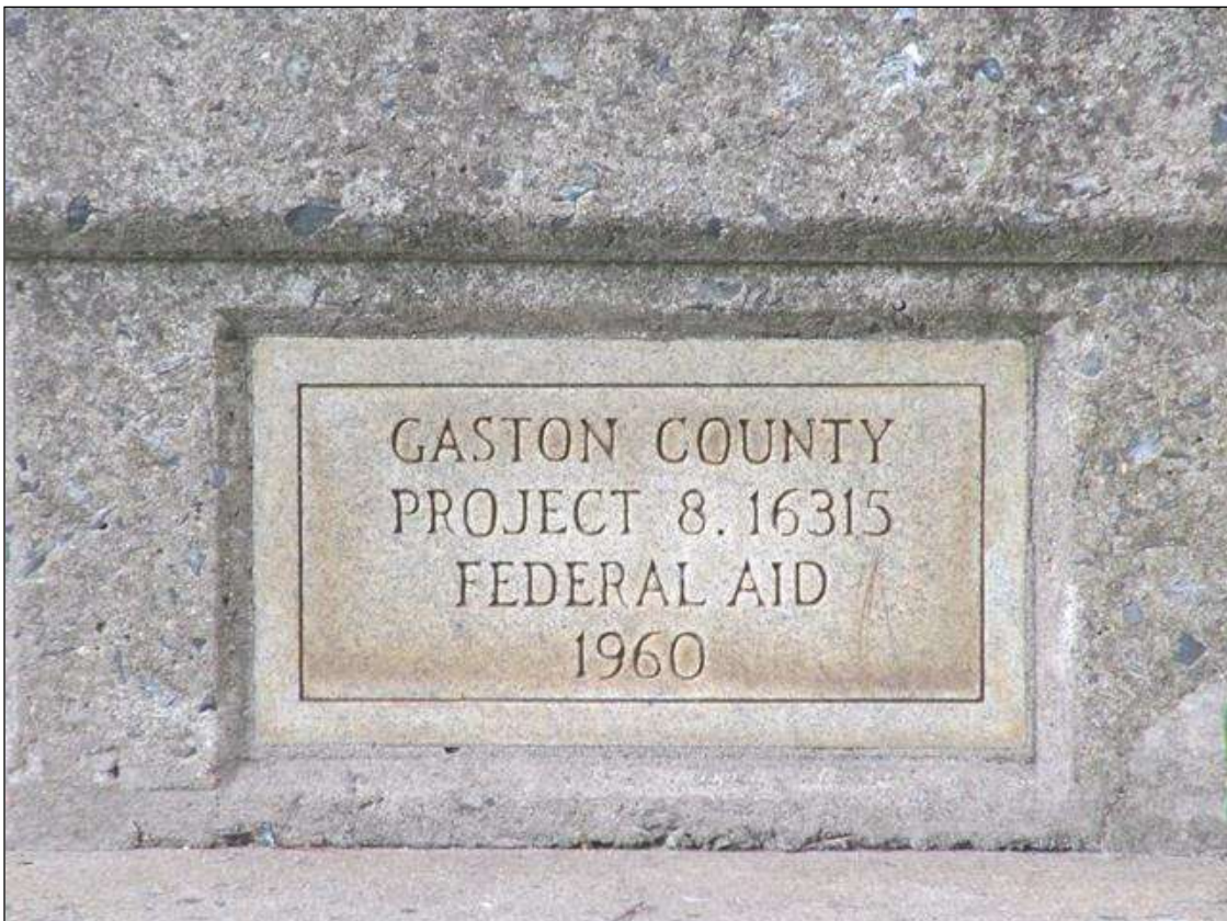
DATA PLATE, NORTHEAST CORNER
