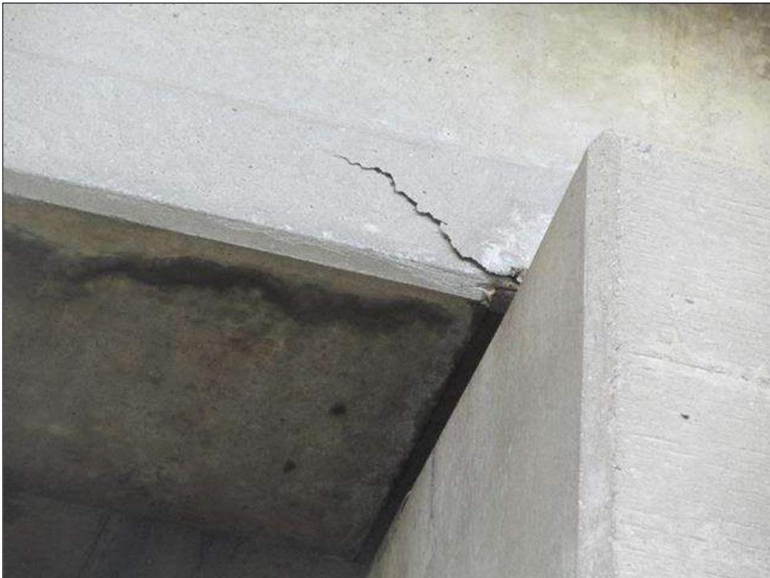
CRACKING IN BEAM 1 END OVER BENT 2, SPAN 3. APPROX 2SF
