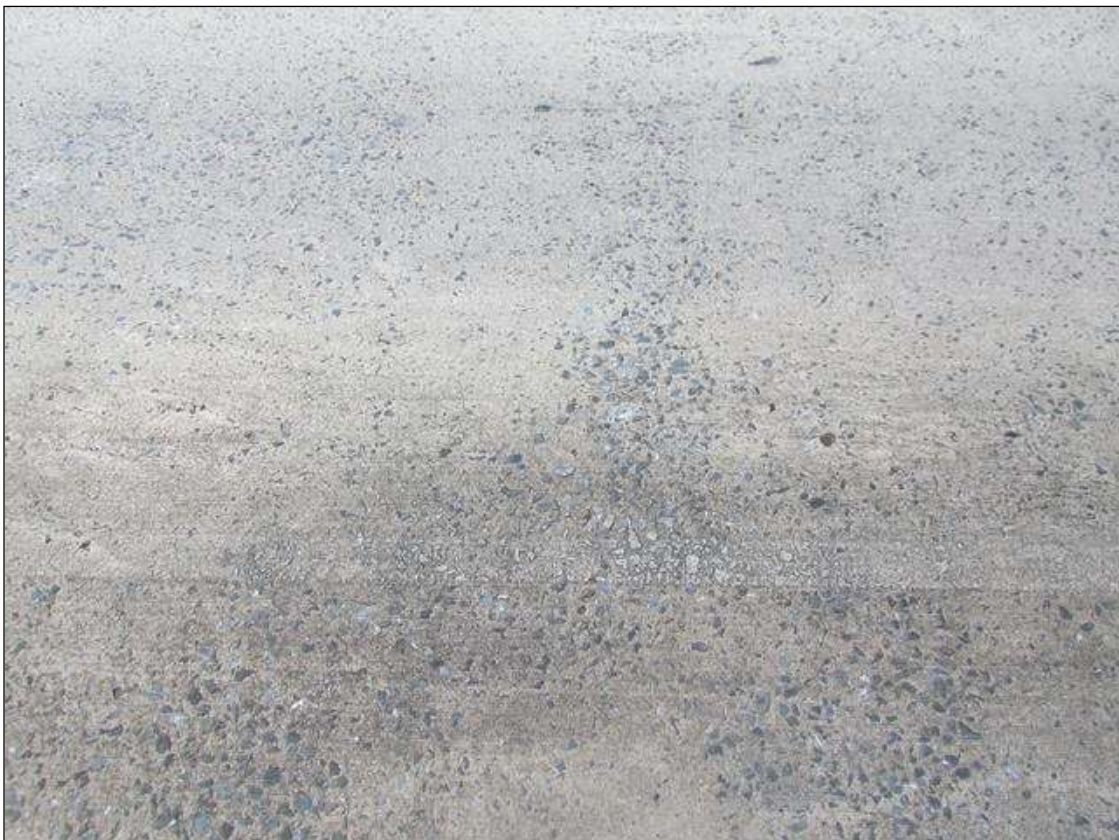
SCATTERED COARSE AGGREGATE EXPOSURE IN TOP OF RC DECK
