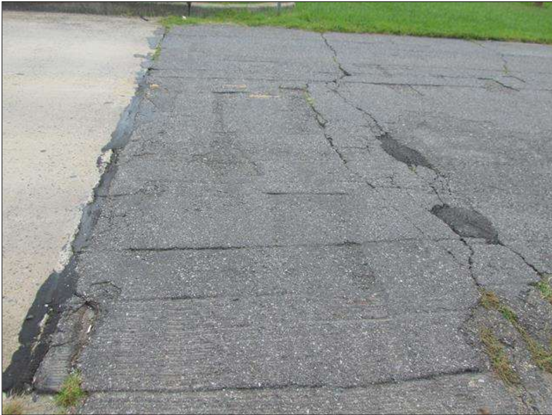
WEST APPROACH HEAVED, CRACKED, AND POTHOLING.
