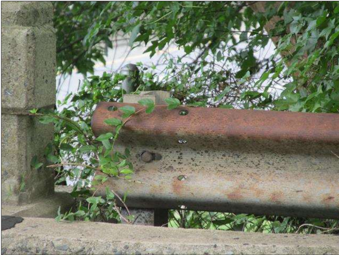
GR NOT ATTACHED, NORTHEAST CORNER
