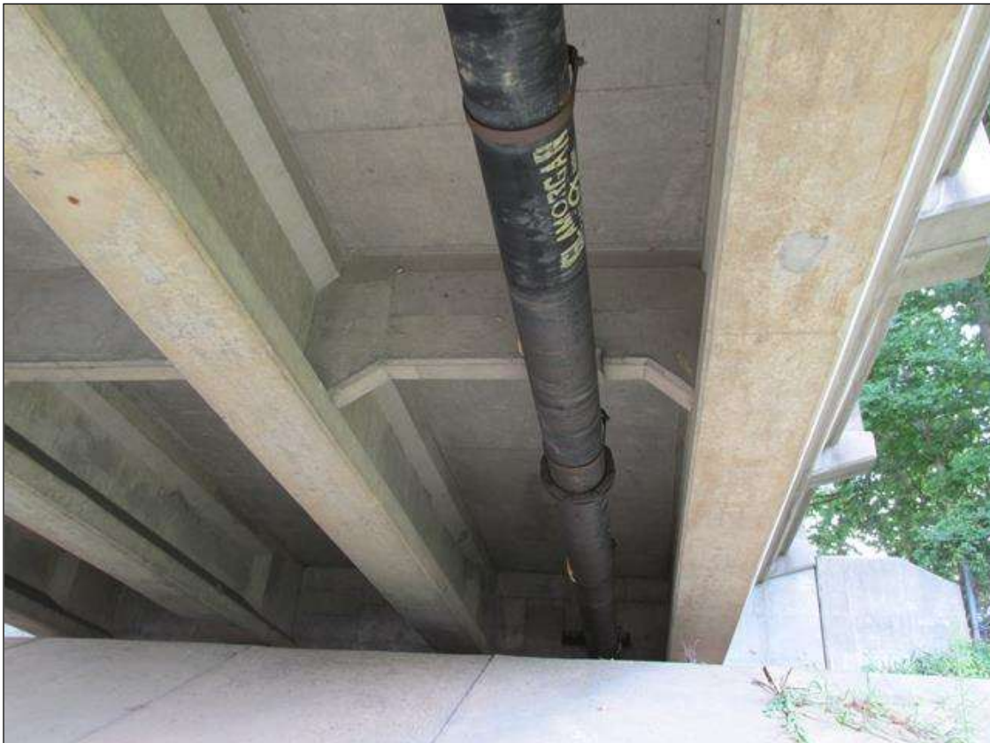
12" DIP HANGING FROM STEEL SUPPORTS IN BAY 3
