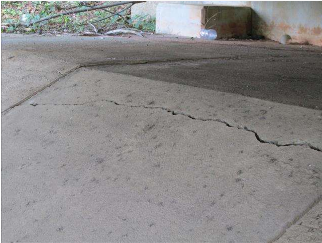
SCATTERED CRACKING IN POURED CONCRETE SLOPE PROTECTION
