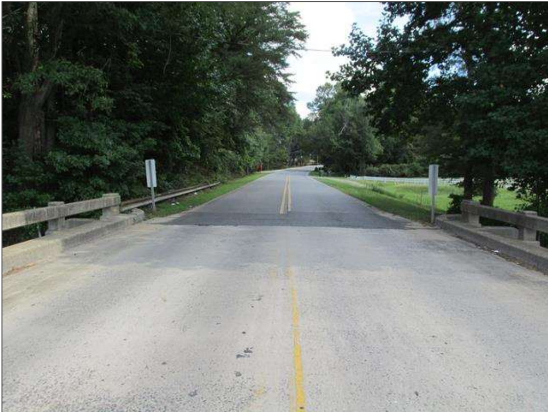
GUARDRAIL LOOKING EAST
