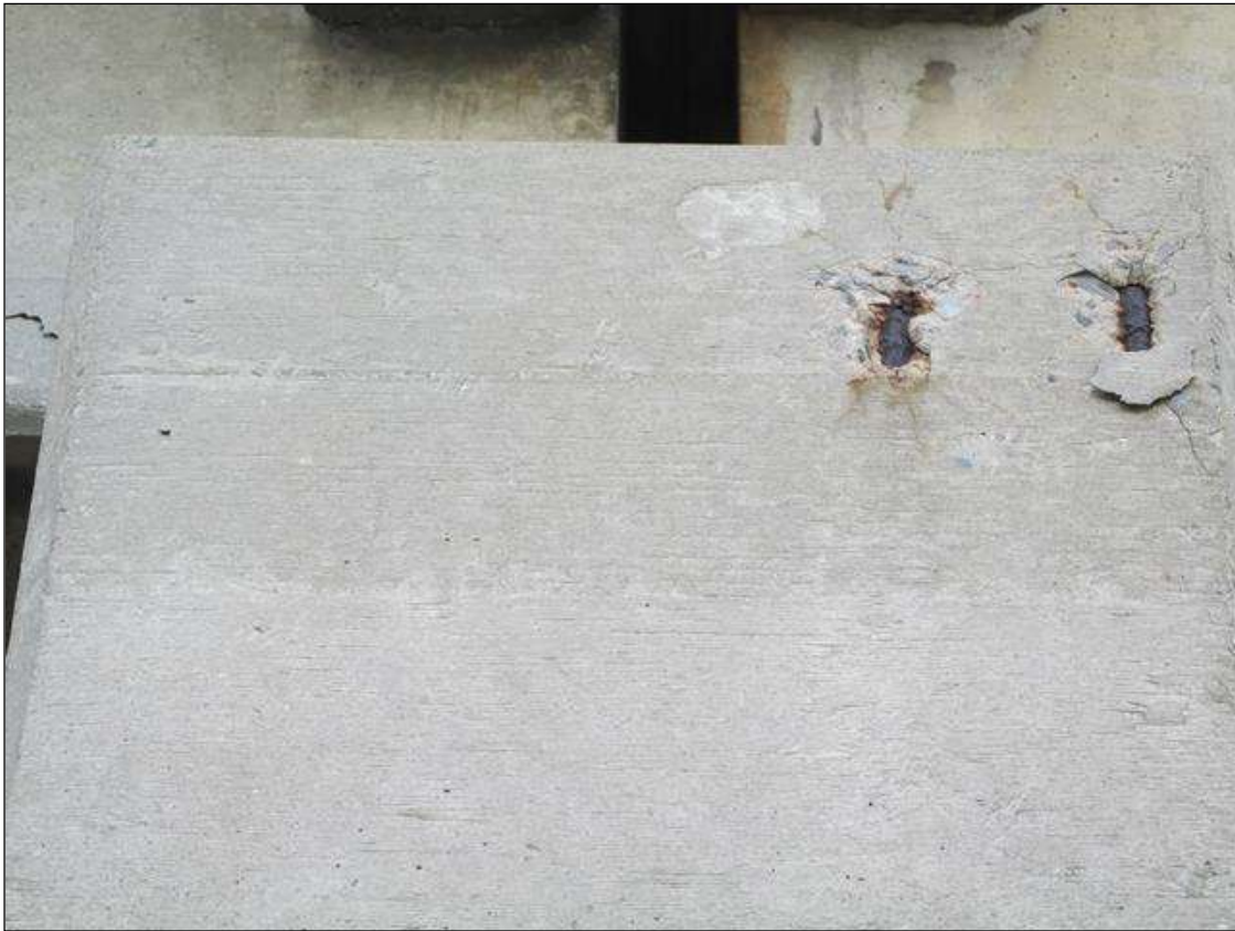
SPALLING WITH RESTEEL EXPOSED ON SOUTH END OF BENT 2 CAP, APPROX 2SF.
