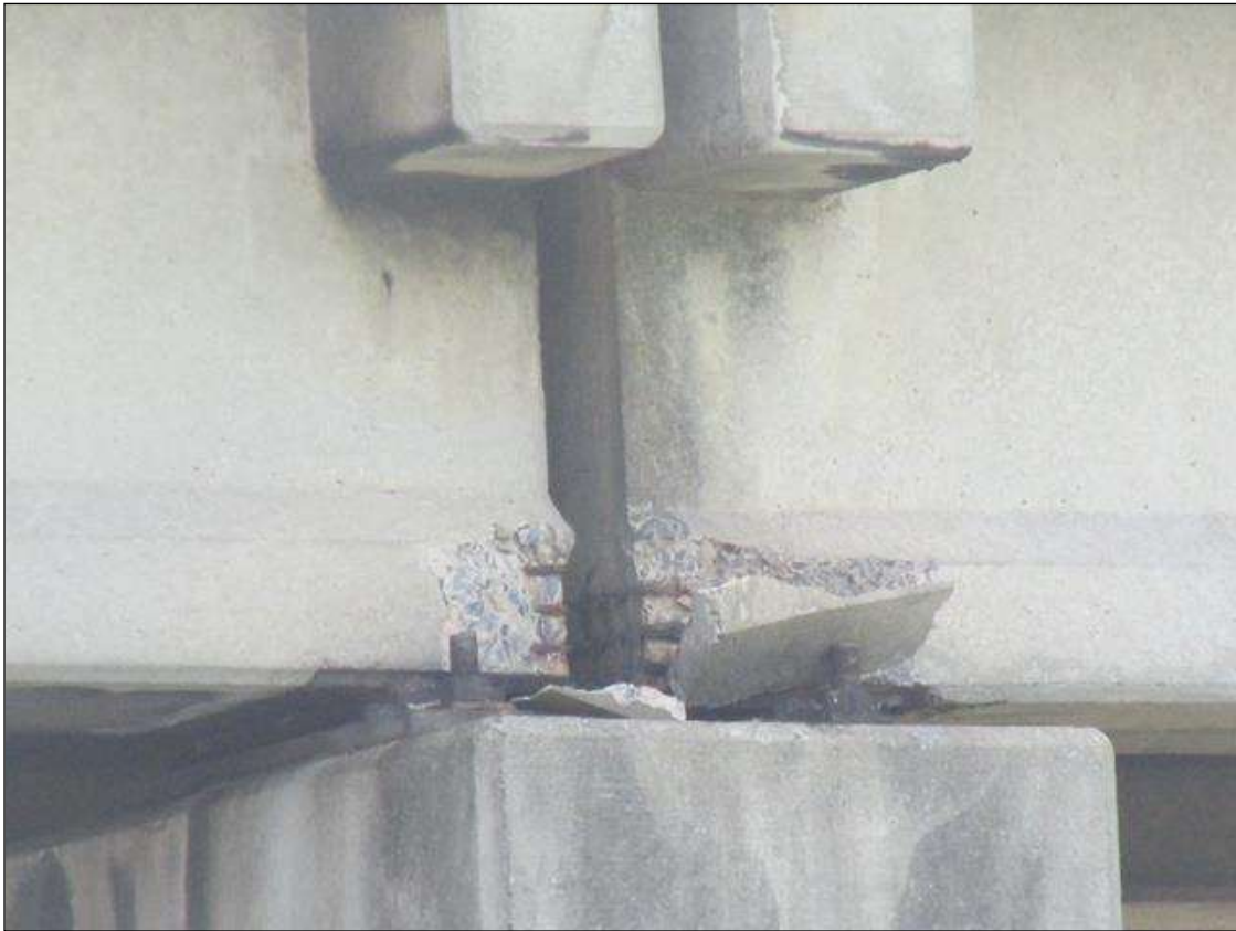
SPALLING IN BEAM ENDS WITH RESTEEL EXPOSED, OVER BENT 1, BEAM1 IN SPANS 1 AND 2.
