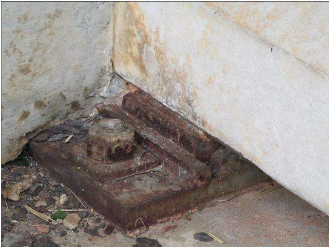
SCATTERED SURFACE CORROSION ON BEARINGS THROUGHOUT SUPERSTRUCTURE, CONCENTRATED AT BENTS.
